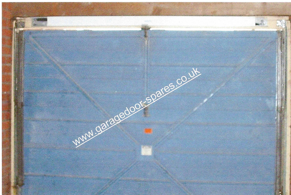
The New Spring Box Fitted
